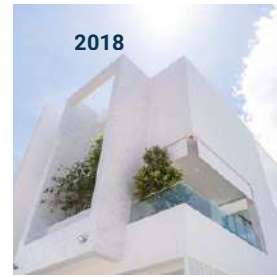
THE RESIDENCE BY ANDAMAN ASSET SOLUTION
